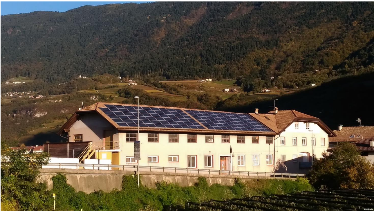
Fig.19 (Solar roof in Salerno, Alto Adige, Italy)
