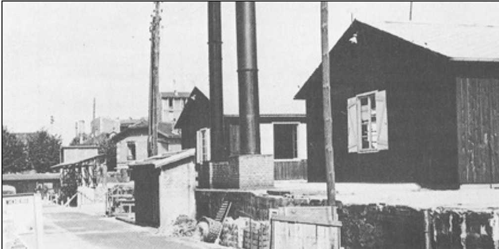
Photo from 1948 showing CNET-SRCT buildings in the suburb of Paris illustrating the adverse situation in France immediately post-war [DUP 07]
